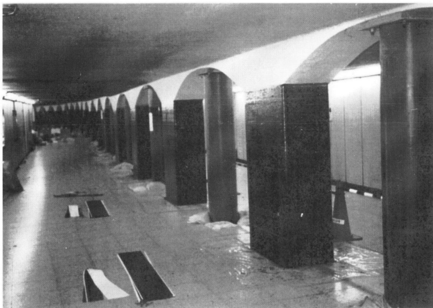
Figure 24. Seismic retrofit of railway station's columns.
