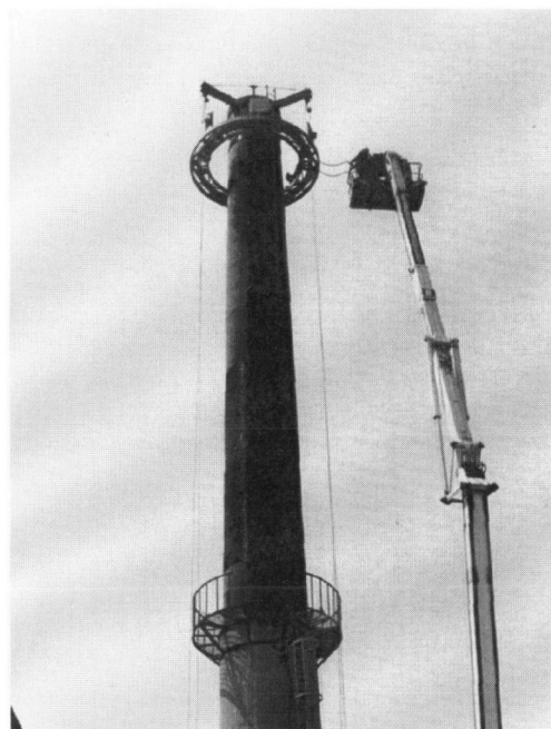
Figure 21. Retrofitting work by automated winding machine for chimney.
