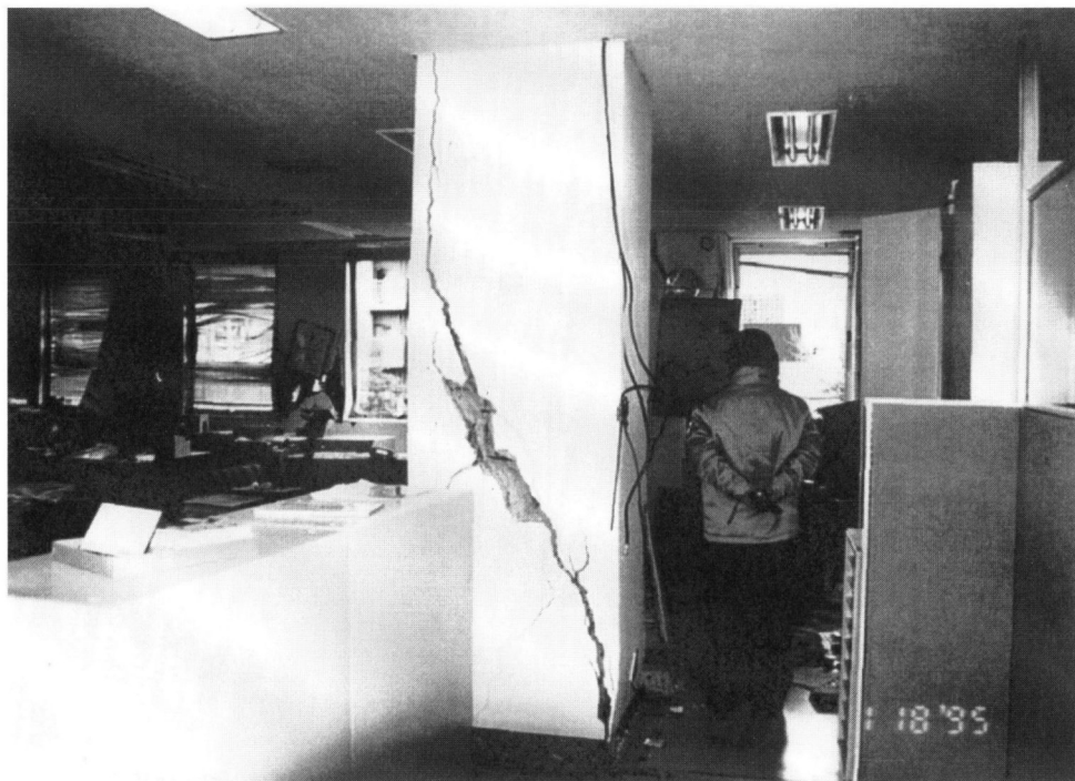
Figure 4. Shear cracks in building column.
