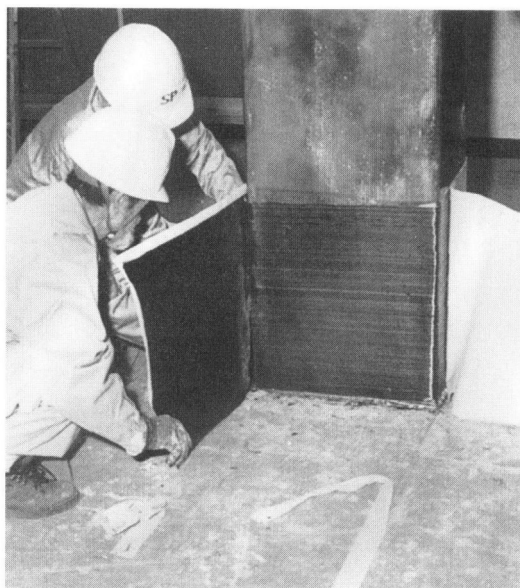
Figure 16. Wrapping work of carbon fiber sheet.
