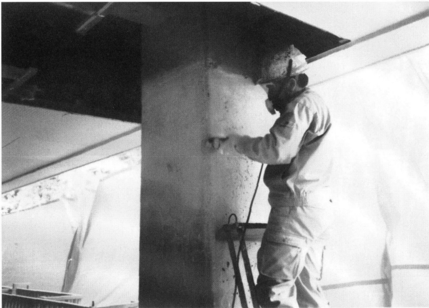
Figure 11. Rounding work of corners.
